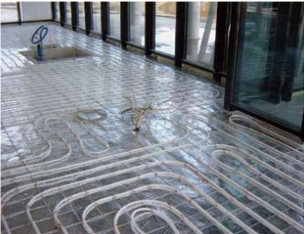
Floor heating on ground floor
